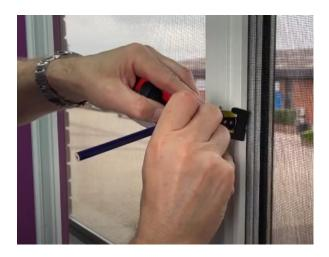
With the screen fully closed, **ensure the central frame is lined up and held firmly in place**. Drill a pilot hole using a 3 ½ mm HSS drill bit first, and then enlarge it using a 6mm HSS bit. Take the holes all the way through both frames to the back.
